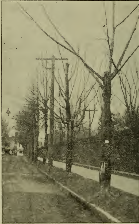
Fig. 24. Showing disfigurement of trees caused by burning from electric wires.
